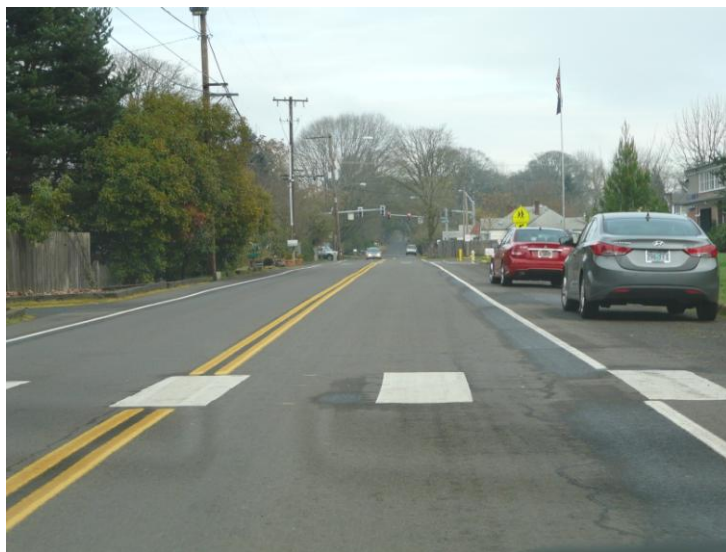
Hilliard Lane Looking East in Front of School
